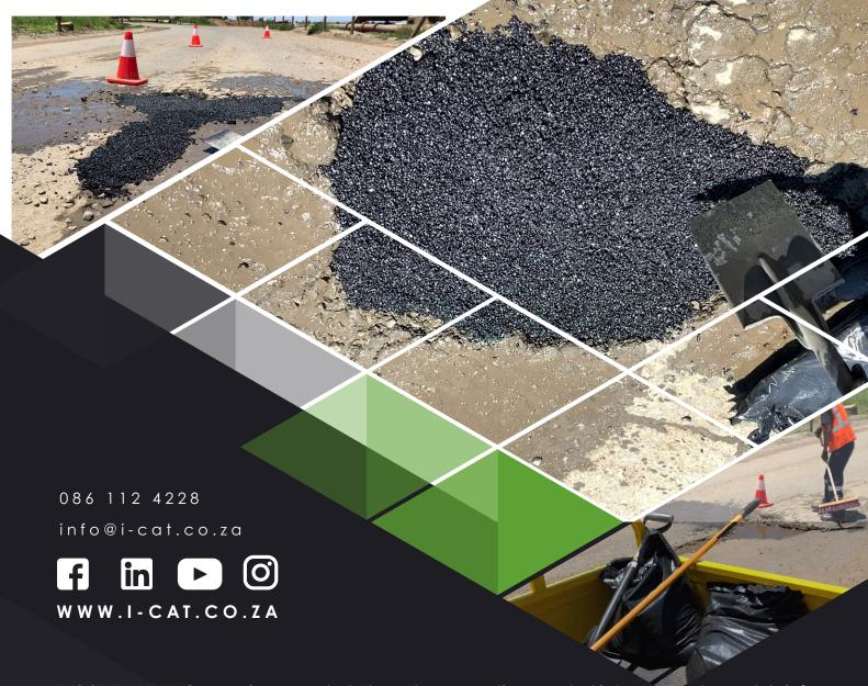
IT IS SELF-PRIMING: No primer needed. The only preparation needed is to remove loose debris from the pothole prior to filling.
